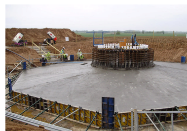
Turbine foundation under construction
