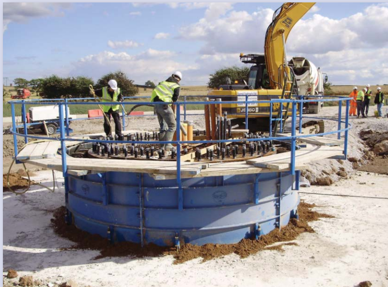
Completing the collar at T7 to which the turbine tower will be bolted.
