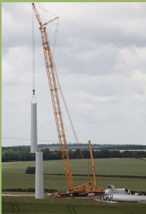
1. The tower sections are connected together.
